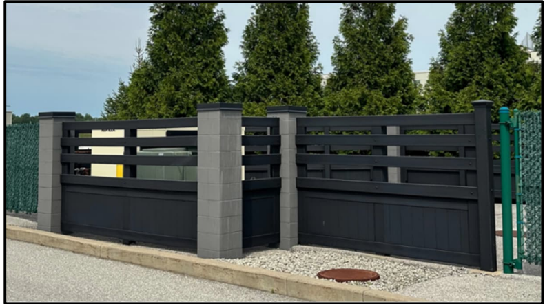
Figure 6: Example of existing onsite screening
